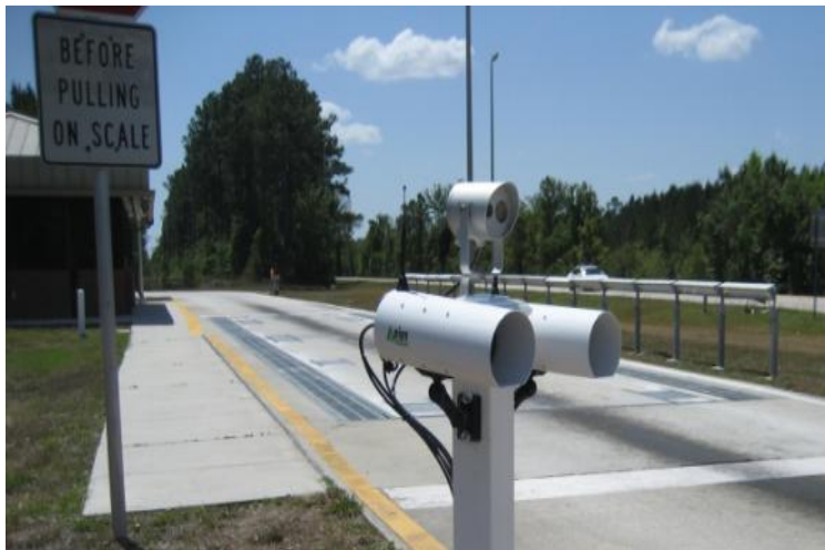
ALPR camera in use at a roadside truck scale
